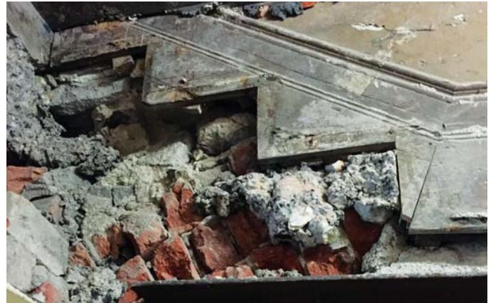
*Degradation of masonry and plaster due to moisture*
